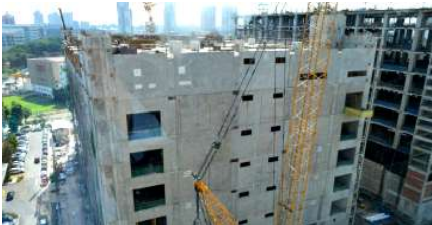
Roof construction in-progress
